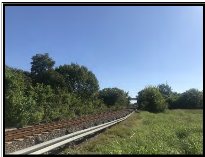
RR track along the subject's northern boundary
