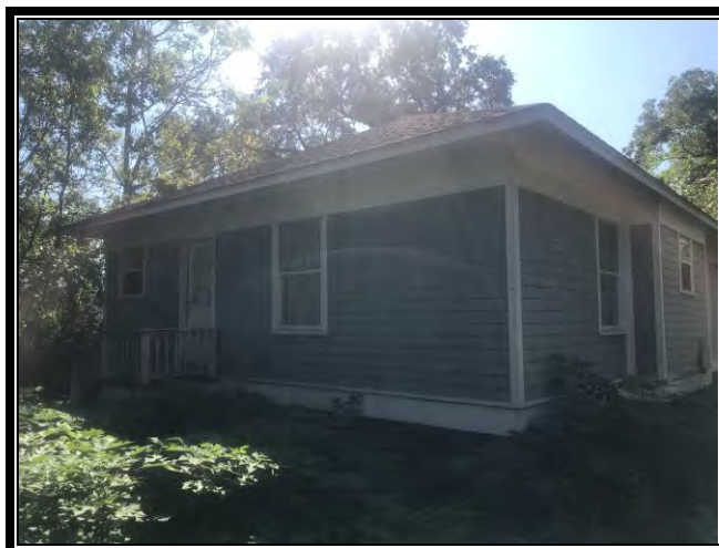
View of back of house on subject property
