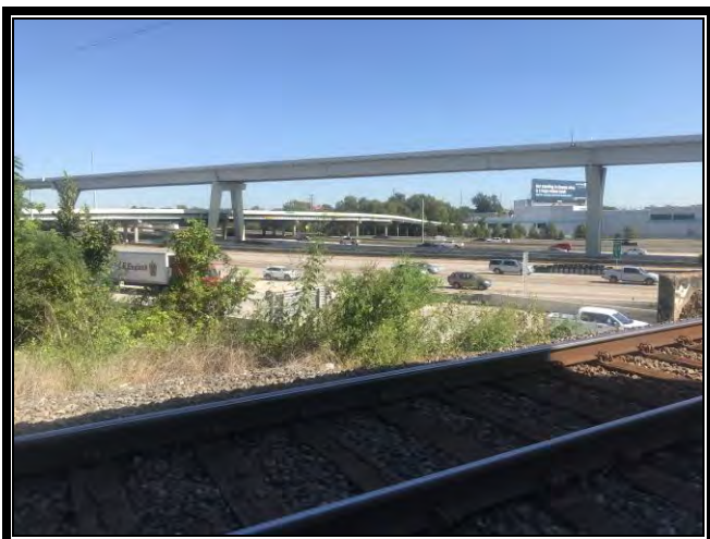
View of I-45/I-10 as seen from RR track
