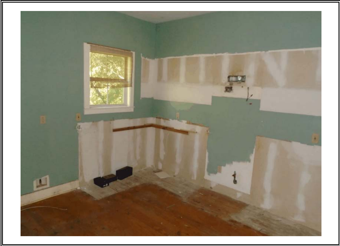
View of Kitchen Area
